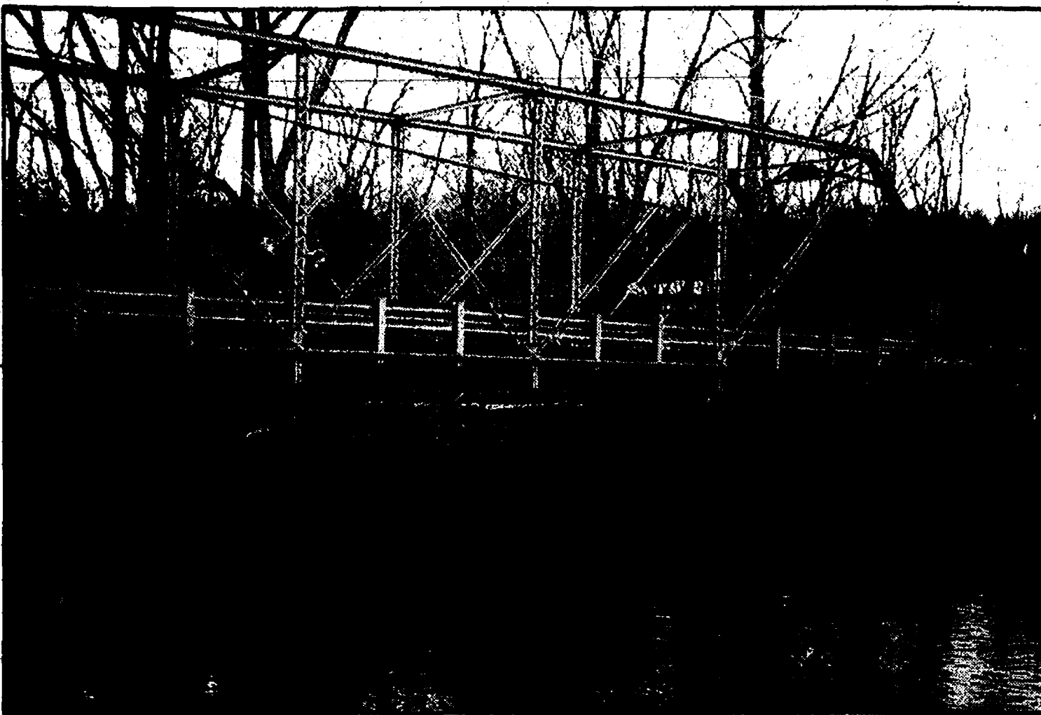
THE BELL ROAD BRIDGE in Dexter Township will be the topic of discussion at a meeting slated today at the County Annex Building in Ann Arbor. Residents Janice Schneider and Kathy VanVorhis are rallying their neighbors to help save the bridge. The Washtenaw County Road Commission is considering four outcomes for the bridge's future. Area residents would like the bridge restored.
